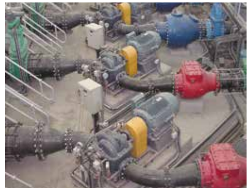
Potable Water Pump CDM400×350mm, 1,620m 3 /h, 35m, 200kW CDM350×300mm, 1,080m 3 /h, 35m, 150kW
