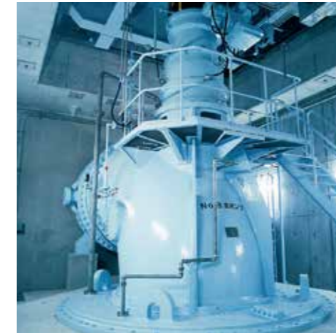
Dewatering pump with adjustable vane (Size:2,400mm, Driver:1,103kW)
