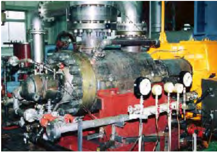
Barrel casing boiler feed pump 2,925psi-2,980 U.S.gpm-5,610min -1 -7,240HP Petacalco Power Plant(Mexico), 350MW×4units
